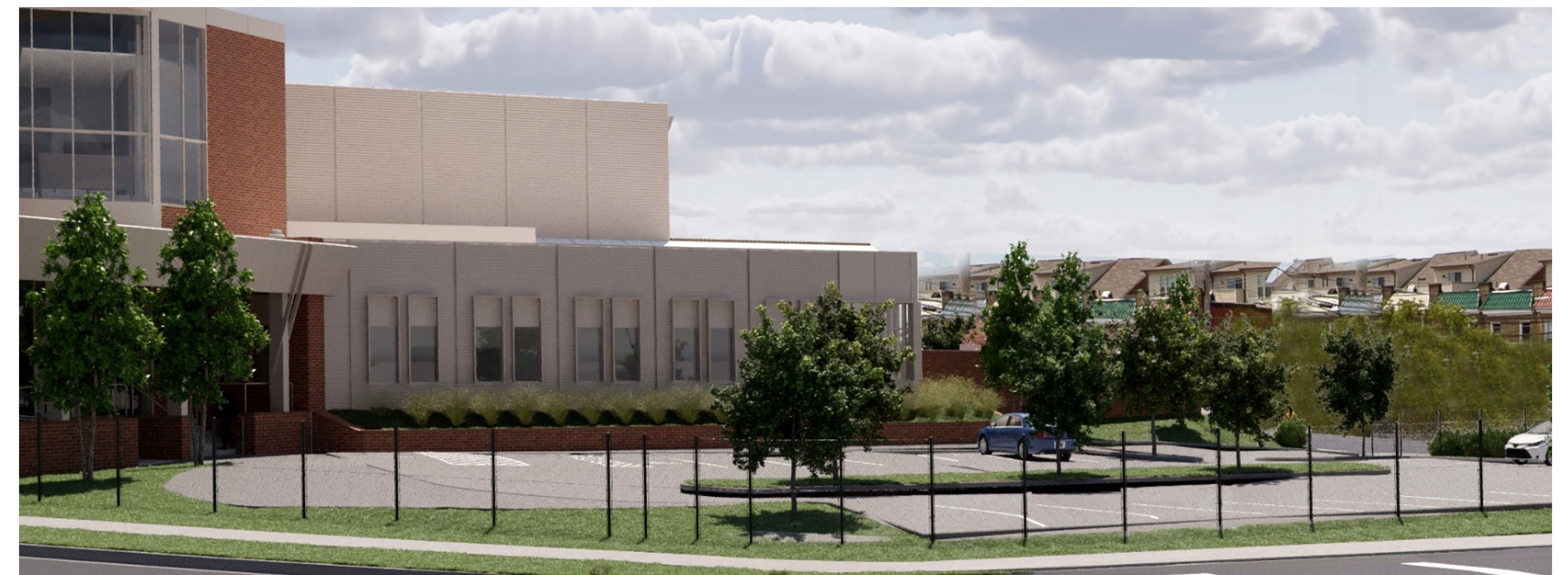
Southwest Facing View – Ponca Street Transportation and Maintenance Building
