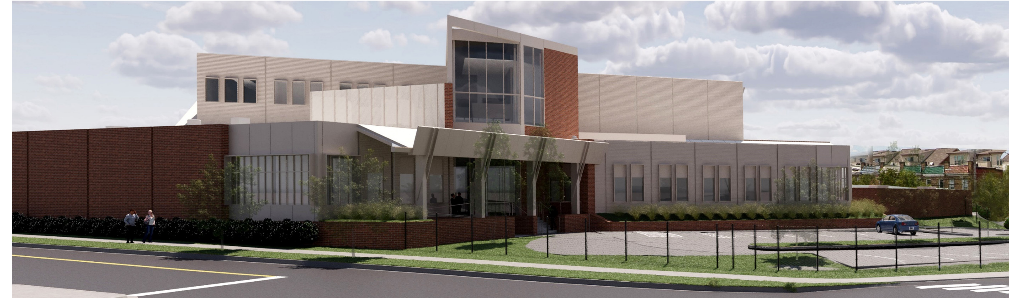
Southwest Facing View – Ponca Street Transportation and Maintenance Building
