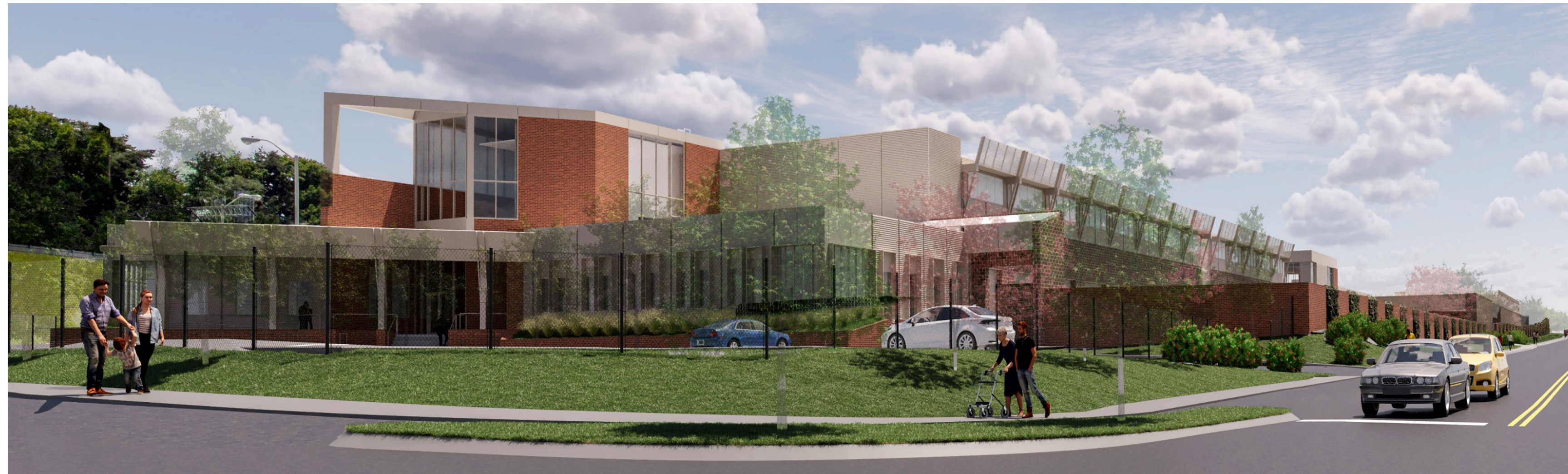
Southeast Facing View – Oldham Street Transportation and Maintenance Building
