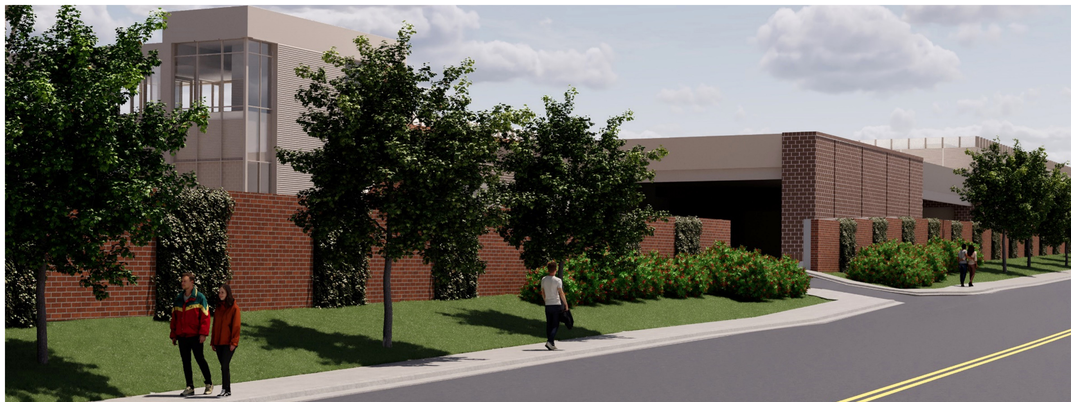
Southeast Facing View – Oldham Street Bus Storage Building
